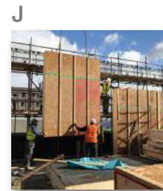
J Panels are joined together to create an air-tight detail and maximise the integrity of the overall structure.
