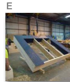
E Panel assembled and closed to one side prior to being flipped over to have straw installed
