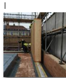
I Panels are located onto a sole plate. This also assists when creating an air-tight seal between the base of the panel
