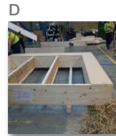
D Panel frames are assembled.
